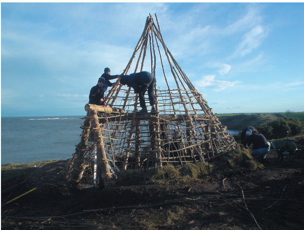
Figure 13.10 The hut begins to take shape as an entrance is attached and the turfing begins.
