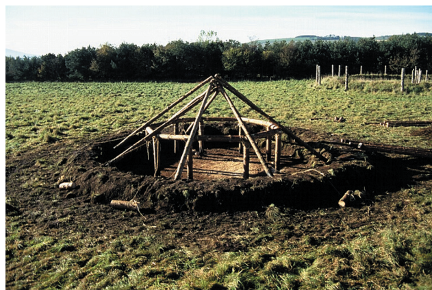
Figure 13.3 The hut after erection of the timber uprights, lintels and roofing poles
