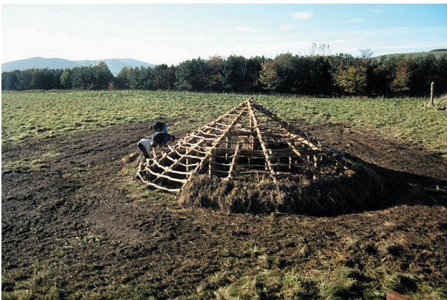
Figure 13.5 Adding the first layer of thatch starting from the base of the roof.
