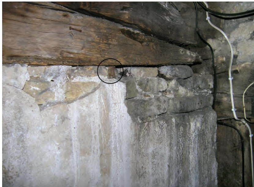
Fig. 7.25: 33 Strand Street (House 83), panel below tiebeam of north truss in hall, with brick filling and short peg or wedge (circled) to hold bricks in place (S. P.)
