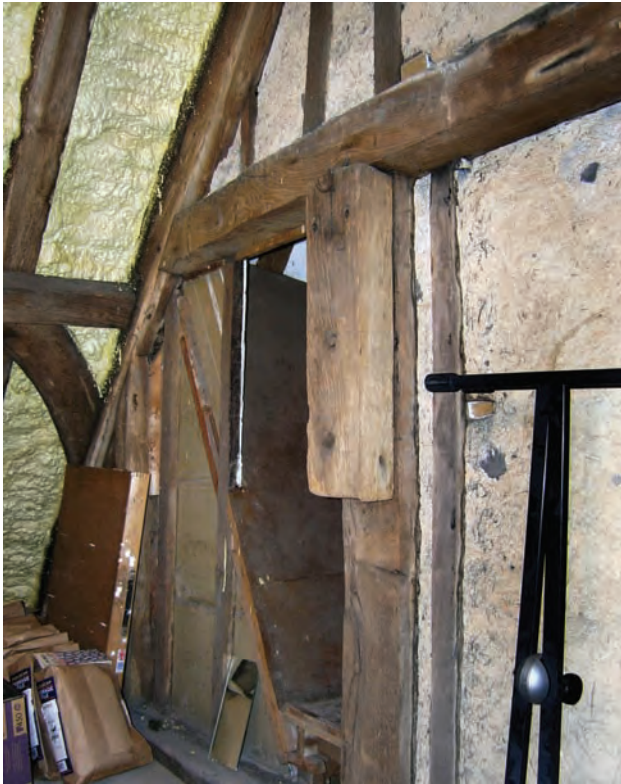
Fig. 12.47: 3 Strand Street (House 74), timber block on street face of closed roof truss at north end of the hall. It is suggested that it was put here as part of a hoist to draw goods up from the street to the left (S. P.)
