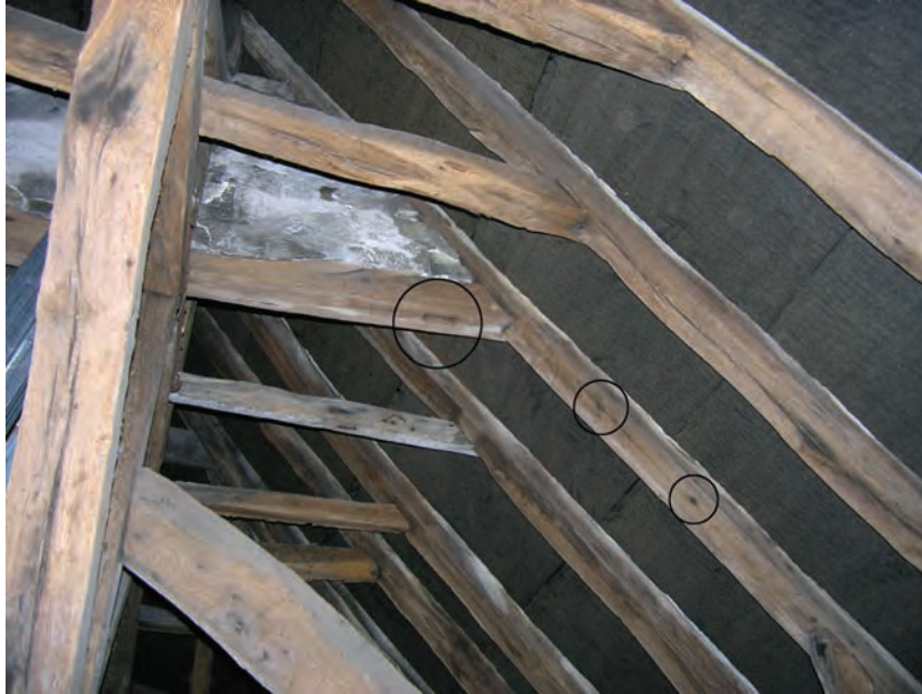
Fig. 7.24: 33 Strand Street (House 83), apex of central closed truss, east range, with brick filling still in place, and mortices (circled) for stud below collar and pegs on rafter, formerly to hold bricks (S. P.)
