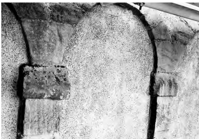
Fig. 261: Tower: Stage 1A, north. Wall-arcading, showing trapezoidal double-springers supported by the plain rectangular capitals of the pilasters. Photo: Warwick Rodwell
