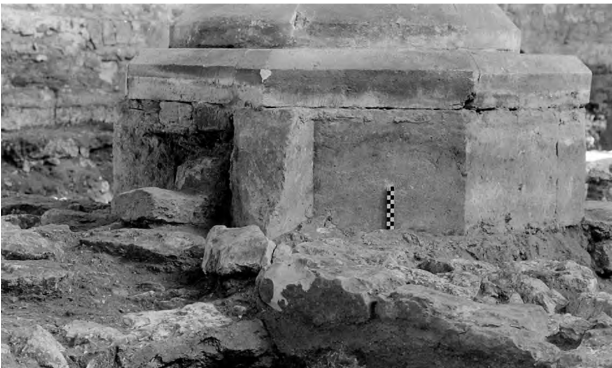
Fig. 488: North arcade. Stub of broken ashlar indicating where the arcade bench in bay 2 was bonded to the plinth of pier 1/2. View north-east. Scale of 10 cm. Photo: Warwick Rodwell
