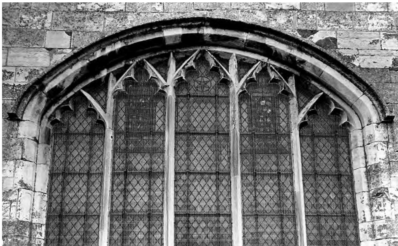
Fig. 559: Chancel east window. Late Perpendicular head and tracery, replacing Decorated tracery. Photo: Warwick Rodwell
