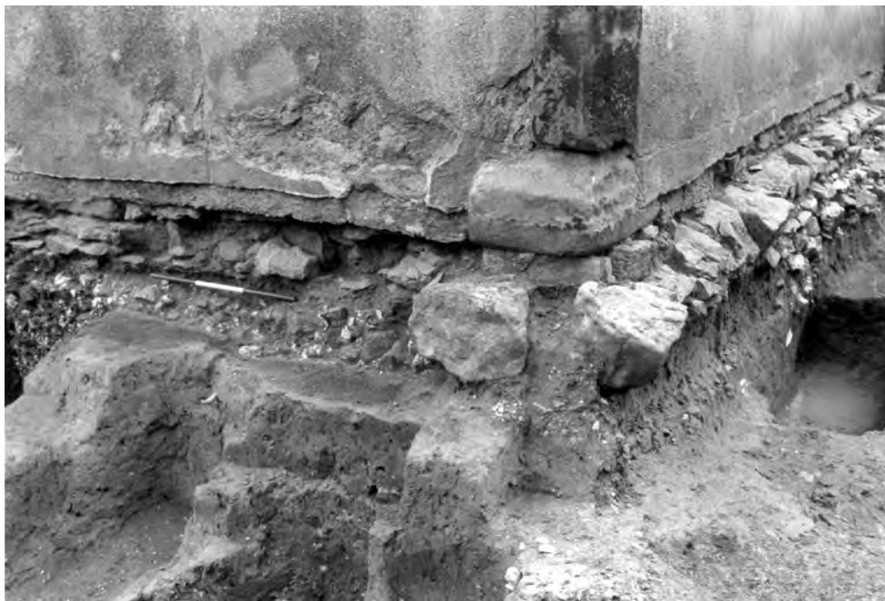
Fig. 326: Western annexe: south-west corner. The limestone plinth running around the base of the walls is present but heavily decayed on the south (right), while on the west (left) it has largely disappeared. Scale of 75 cm. Photo: Warwick Rodwell
