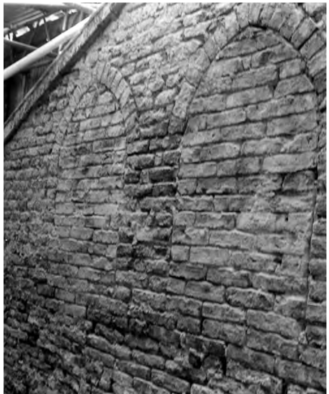
Fig. 590: Nave, exterior of the east gable, 1984. Two blocked openings which formerly ventilated the space between the roof and the ceiling. Photo: Warwick Rodwell
