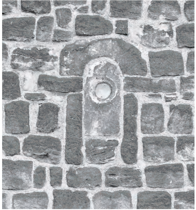
Fig. 292: St Paul, Jarrow (Durham). Monolithic window head formed from a block of Roman masonry. Photo: Warwick Rodwell
