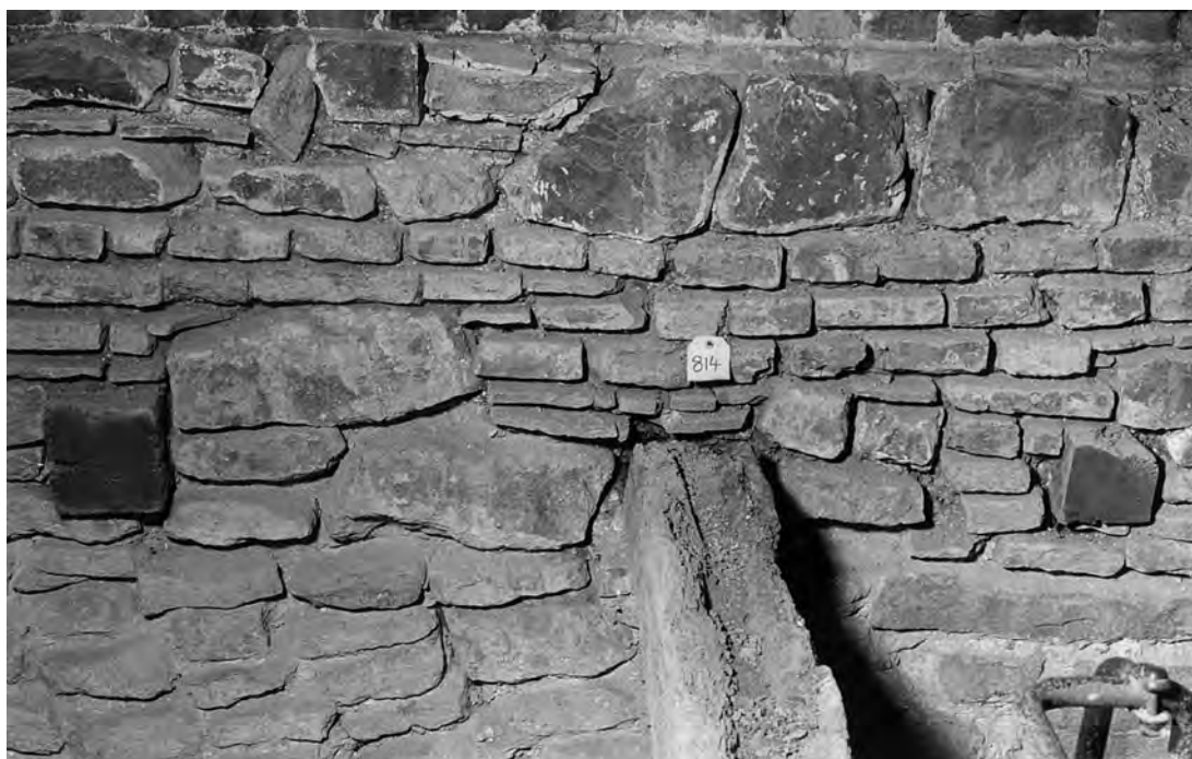
Fig. 329: Western annexe. The top of the north wall, showing one primary floor joist in situ and the stumps of two others that have been sawn off. Photo: Warwick Rodwell
