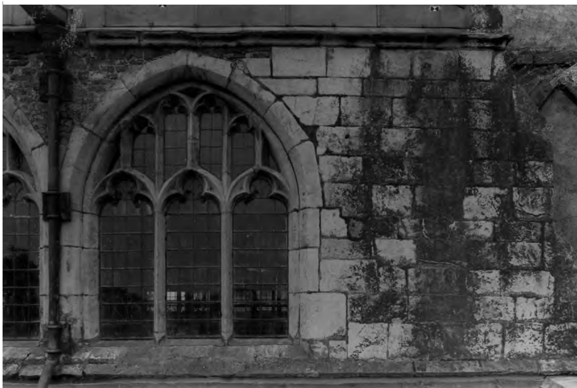
Fig. 542: North clerestory. A, Bay 1 (east); B, Bay 9 (west); showing windows and adjoining nibs of brickwork and ashlar masonry, 1983. Photos: Warwick Rodwell
