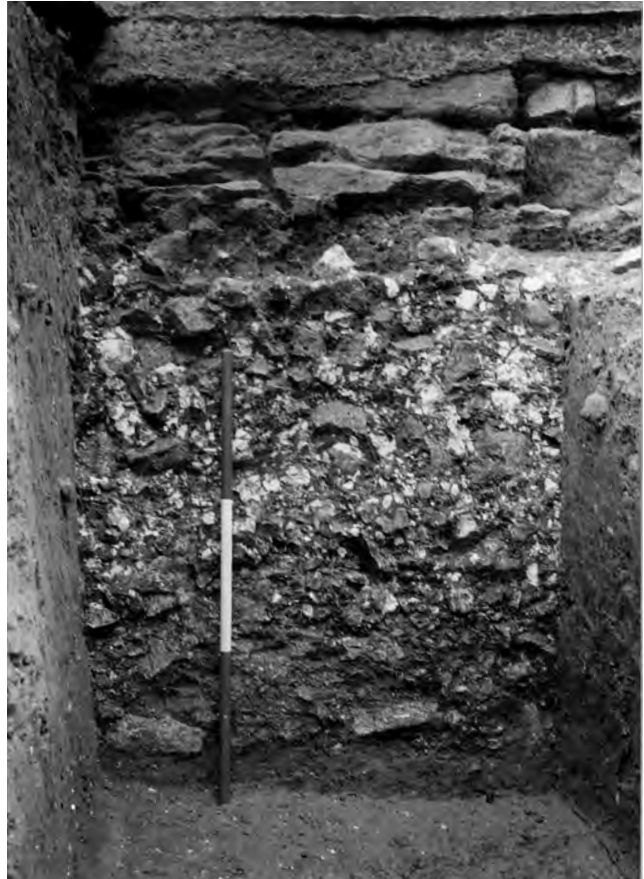
Fig. 303: Western annexe. External face of the rubble foundation on the west side, with the severely fractured limestone plinth course above. Scale of 75 cm. Photo: Warwick Rodwell
