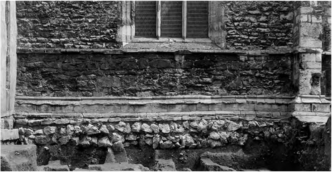
Fig. 440: South aisle, Period 5: west wall. Thirteenth-century chalk rubble foundation, encasing and extending the foundation of the Norman narrow aisle. Note the slightly undulating profile of the plinth, resulting from subsidence. Photo: Warwick Rodwell
