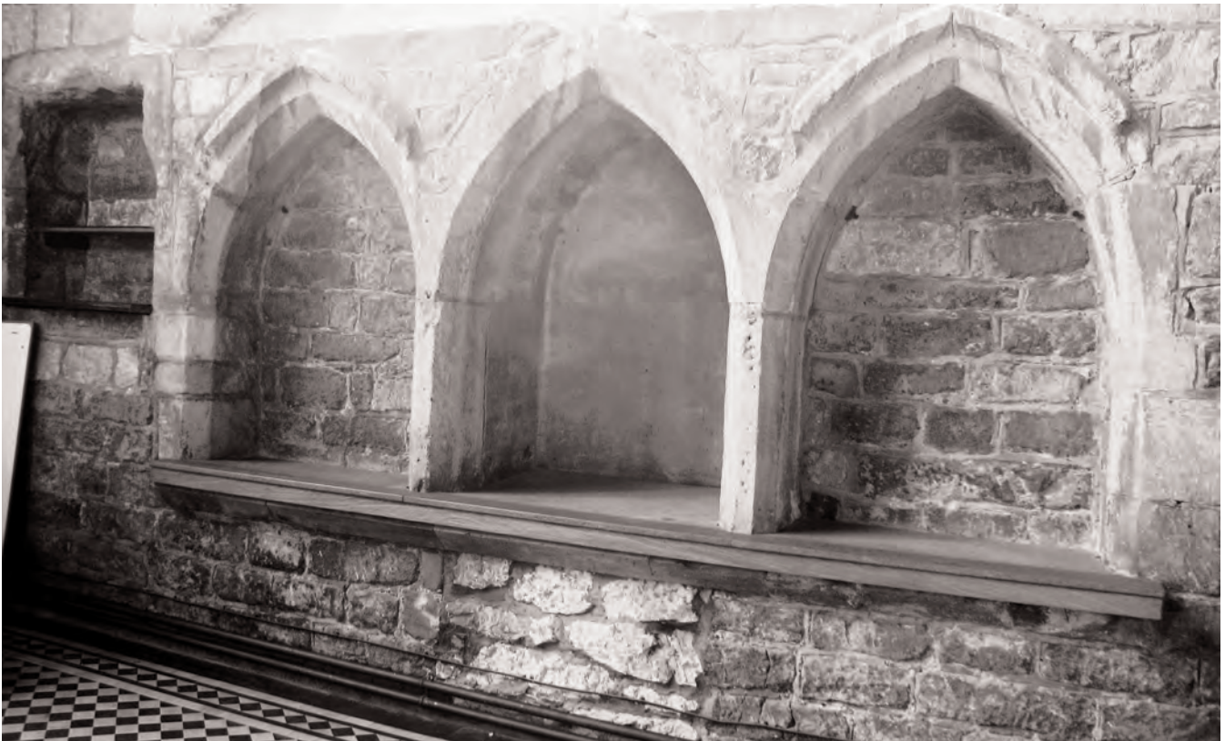
Fig. 59: St Mary's: south chancel aisle. Piscina and sedilia in south wall, the central seat restored after being converted into a doorway. Photo: Warwick Rodwell
