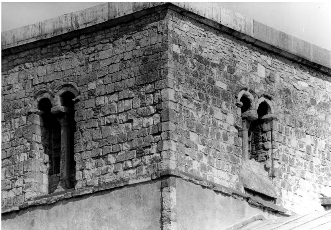
Fig. 399: Tower: Stage 3, belfry. View from the south-east, showing the ashlar masonry construction. Photo: Warwick Rodwell
