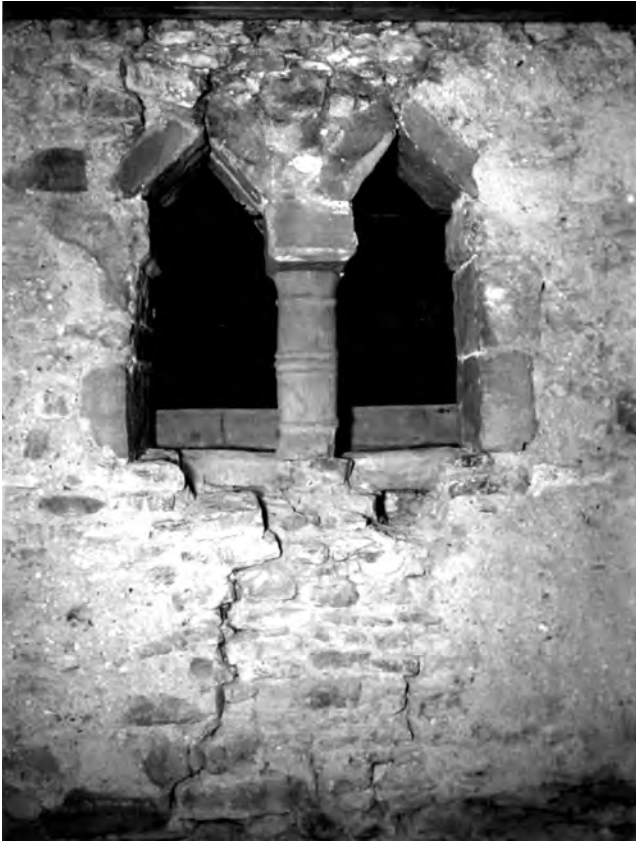
Fig. 299: Tower: Stage 2, interior. East belfry opening, 1983. Note also the cracks in the masonry above and below. Photo: Warwick Rodwell
