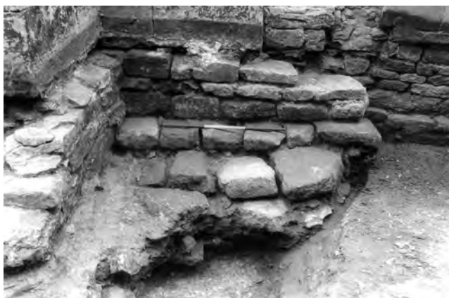
Fig. 446: Chancel: north-east corner. Foundation for a thirteenth-century north-facing buttress, oversailed (top right) by the fourteenth-century east wall of the vestry. View west. Scale of 75 cm. Photo: Warwick Rodwell
