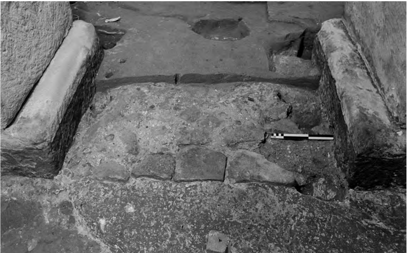
Fig. 317: Tower: threshold of the western arch, edged with flat stones. Overlying the primary lime-concrete surface is an accumulation of grey silty soil. View west. Scale of 25 cm. Photo: Warwick Rodwell
