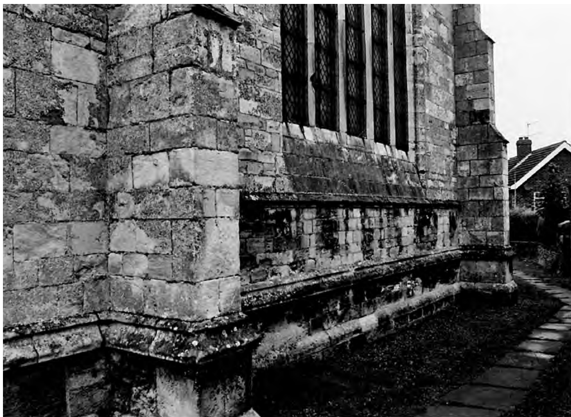
Fig. 534: Chancel. Lower part of the east wall, showing details of the plinth, string-course and raised window sill, 2005. Photo: Warwick Rodwell
