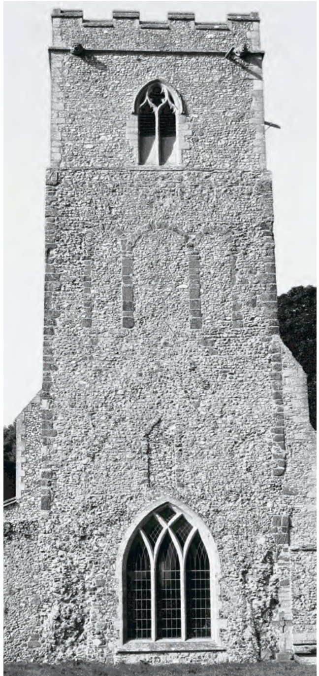
Fig. 369: St Mary, Flitcham (Norf.). East face of the former axial tower, showing the blind arcade of three bays on the third stage. The chancel has been demolished and the window marks the site of the chancel arch; above is a triangular-headed doorway that probably opened from a gallery into a chamber above the chancel. Photo: Warwick Rodwell
