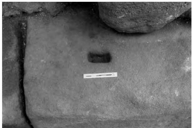
Fig. 305: Tower: details of the plinth at the north-west corner. A, gritstone plinth and fractured base-block of the quoin. B, a small mortice in one of the plinth blocks on the north. Photos: Warwick Rodwell
