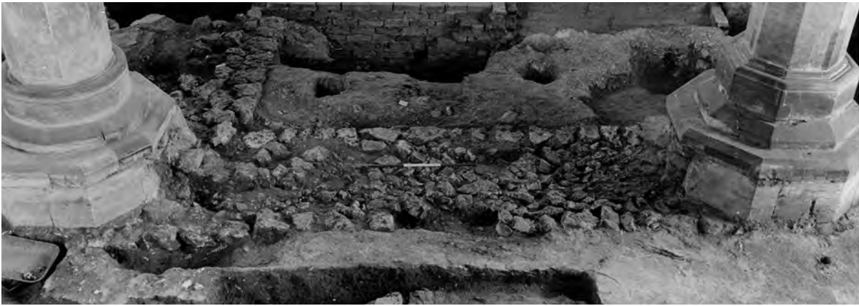
Fig. 487: North arcade, bay 4. The top of the Norman sleeper-wall upon which an arcade bench had been constructed; the latter now entirely destroyed except for scarring on the faces of the plinths of piers 3/4 and 4/5. View south. Scale of 75 cm. Photo: Warwick Rodwell
