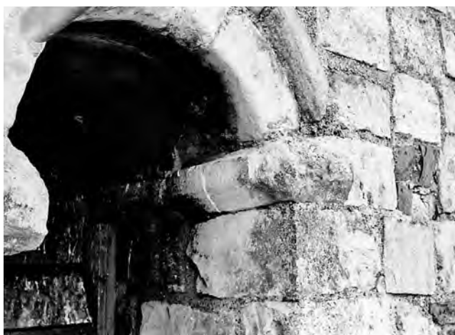
Fig. 403: Tower: Stage 3, southern belfry openings. Details of the double-chamfered string-course blocks reused as imposts. Upper, western aperture. Lower, eastern aperture. Photos: Warwick Rodwell
