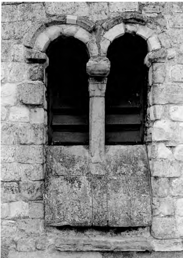
Fig. 409: Tower: Stage 3, east face. Double belfry-opening with later raised sill. Photo: Warwick Rodwell
