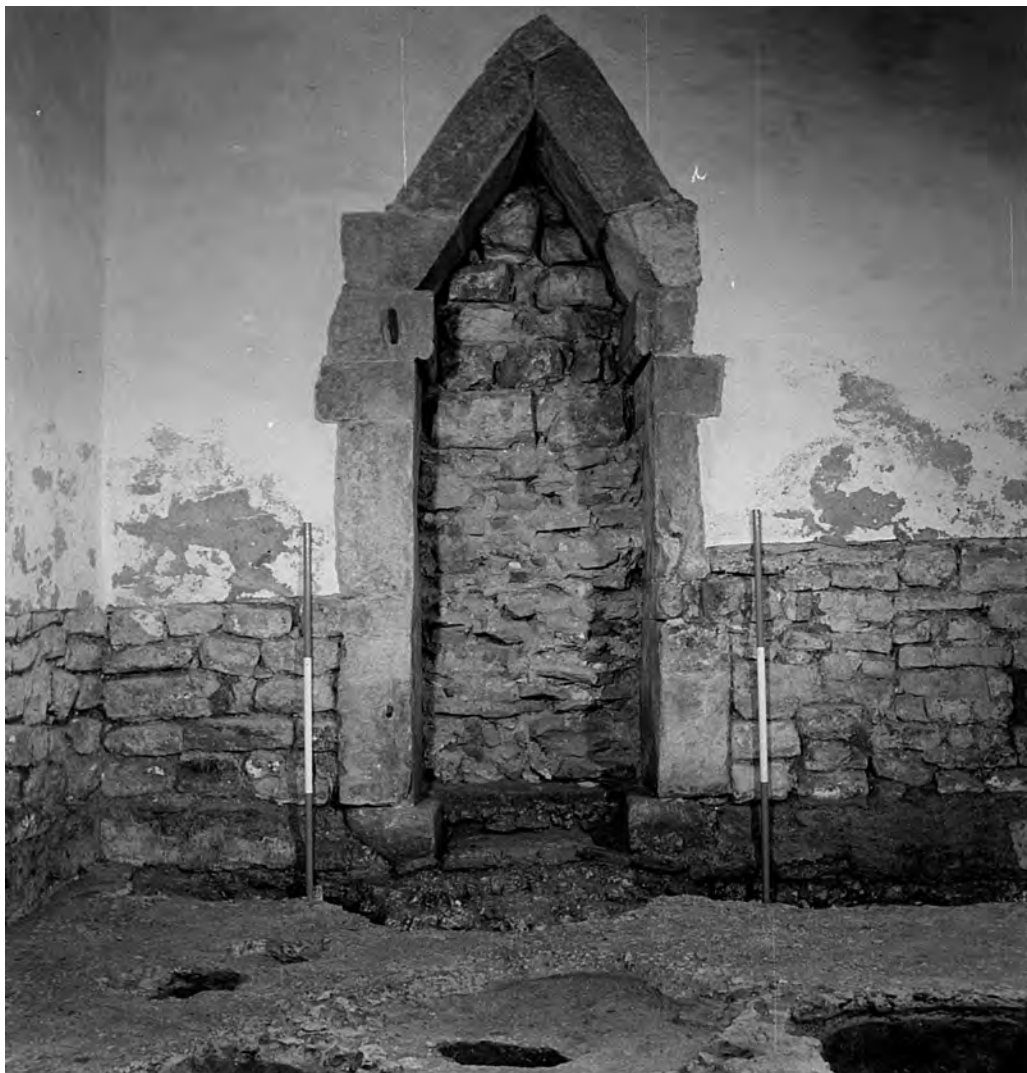
Fig. 321: Tower: north doorway. The 2 m ranging-poles mark the positions of the postholes for a portal-frame flanking the opening. Photo: Warwick Rodwell
