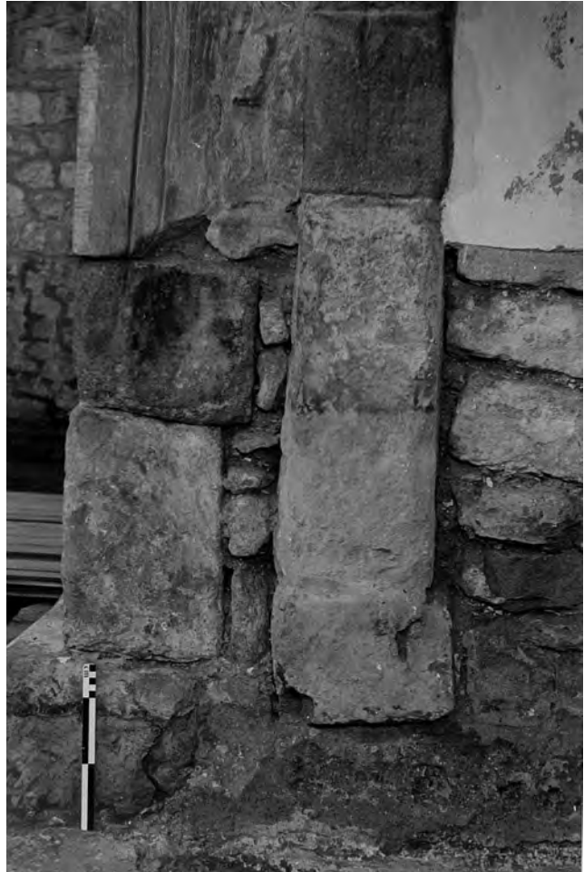
Fig. 283: Tower: Stage 1A. Detail of the base of the south-flanking pilaster-strip of the eastern arch. Note the horizontal line on the first upright stone of the pilaster, defining the pre-1912 floor level in the tower; the burning and consequent decay of the small block in the arch reveal; and the vertical implement-sharpening marks on the stone above. Scale of 25 cm. Photo: Warwick Rodwell
