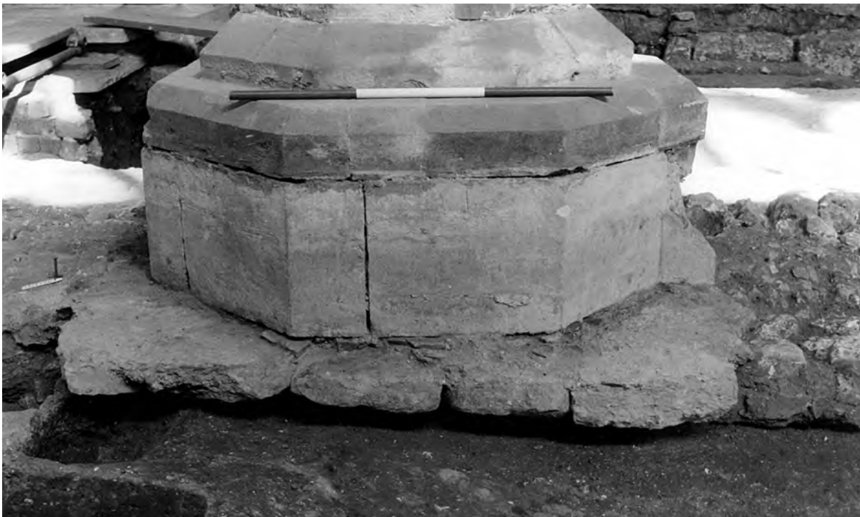
Fig. 482: North arcade. Pier base 4/5 with its shallow footing resting on the Saxo-Norman nave foundation. View north. Scale of 75 cm. Photo: Warwick Rodwell
