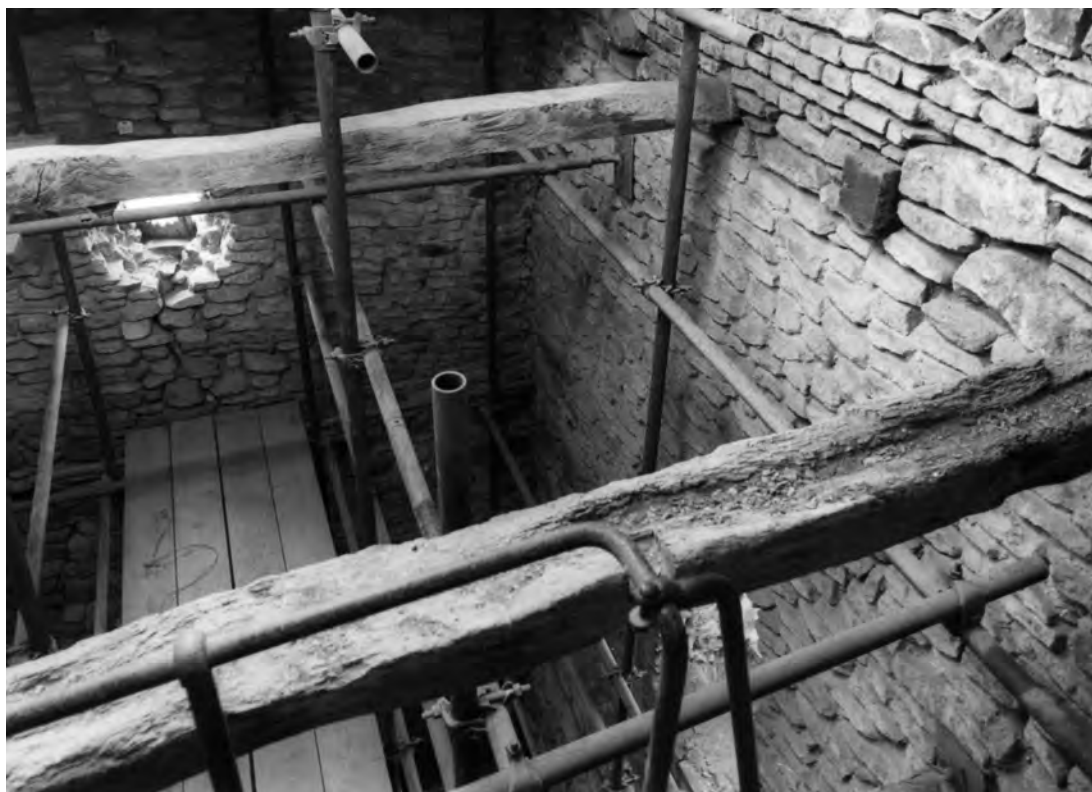
Fig. 328: Western annexe: the upper part of the north wall, showing two existing floor joists (the nearer one being primary) and the sawn-off stump of a third in between. View north-west, 1983. Photo: English Heritage
