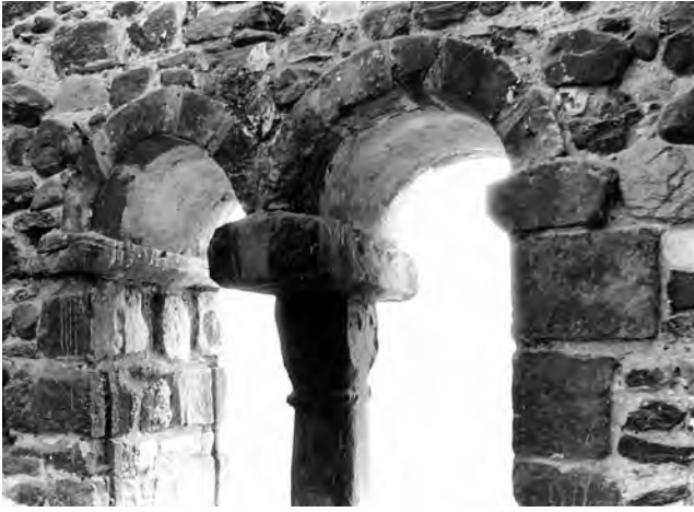
Fig. 412: Tower: Stage 3, interior. Detail of the neatly cut voussoirs in the head of the north belfry opening, 1980. Photo: Warwick Rodwell
