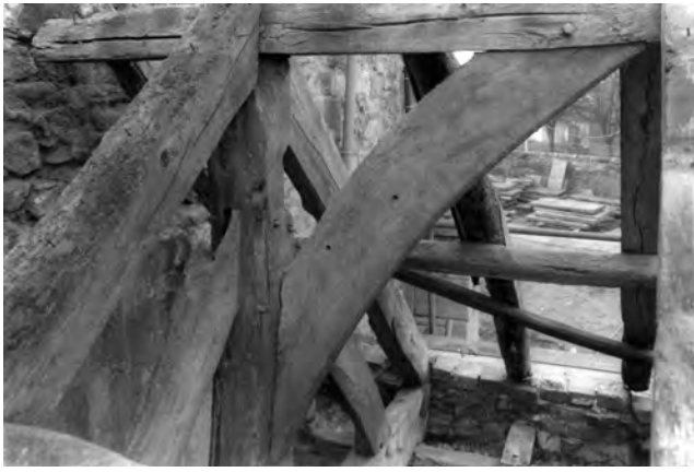
Fig. 555: North porch roof. Detail of the crown-post truss, from the north-east. Photo: Warwick Rodwell
