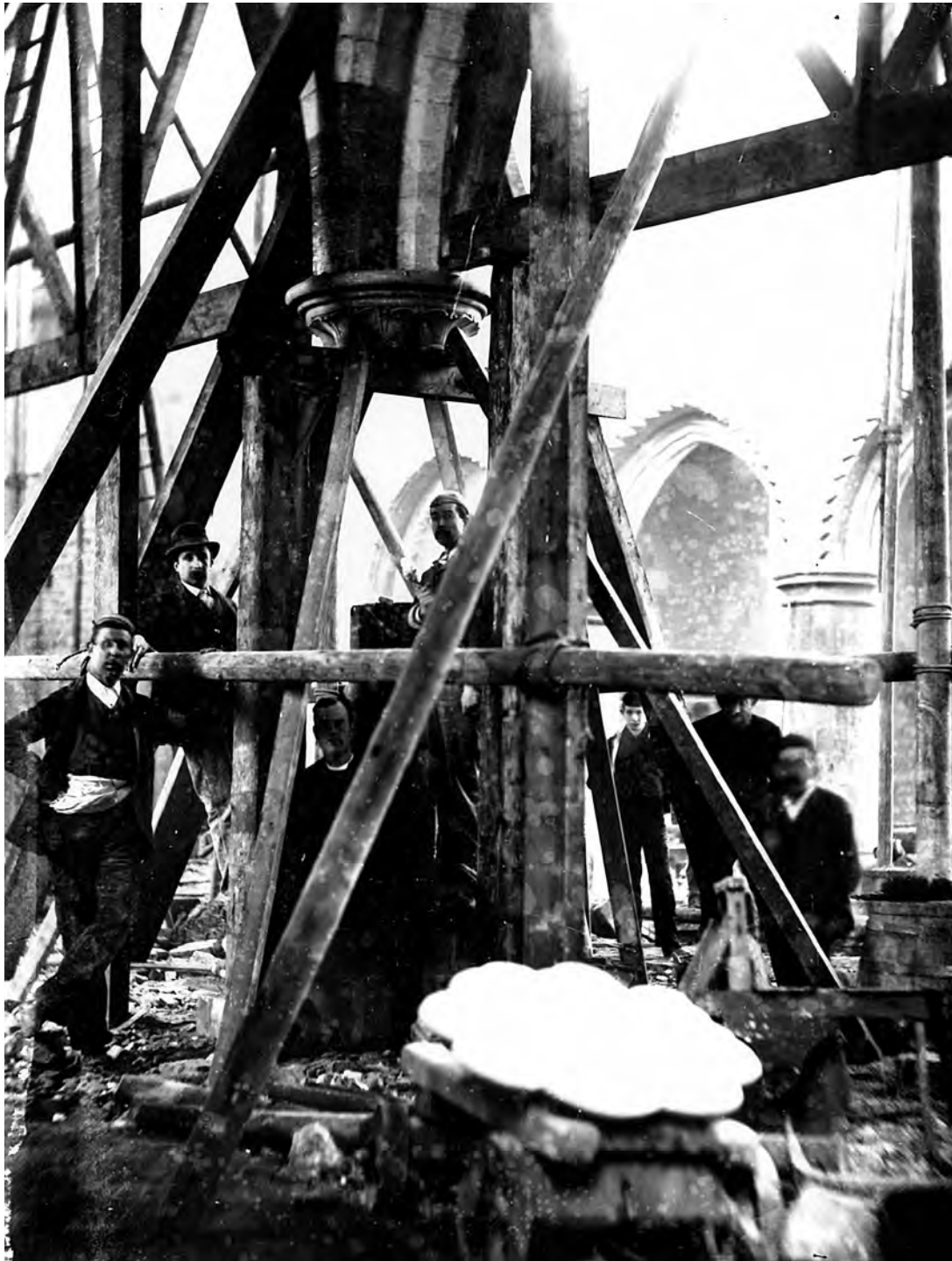
Fig. 71: St Mary's: south nave arcade, 19th January 1892. Shoring in bays 1 and 2, supporting the arches while the pier was entirely removed and rebuilt. Lying on the truck in the foreground appears to be a template for the octofoil base, and sitting under the capital of the removed pier is the vicar, Charles Moor. View north-west. Photo: Arthur Brummitt, courtesy of John French
