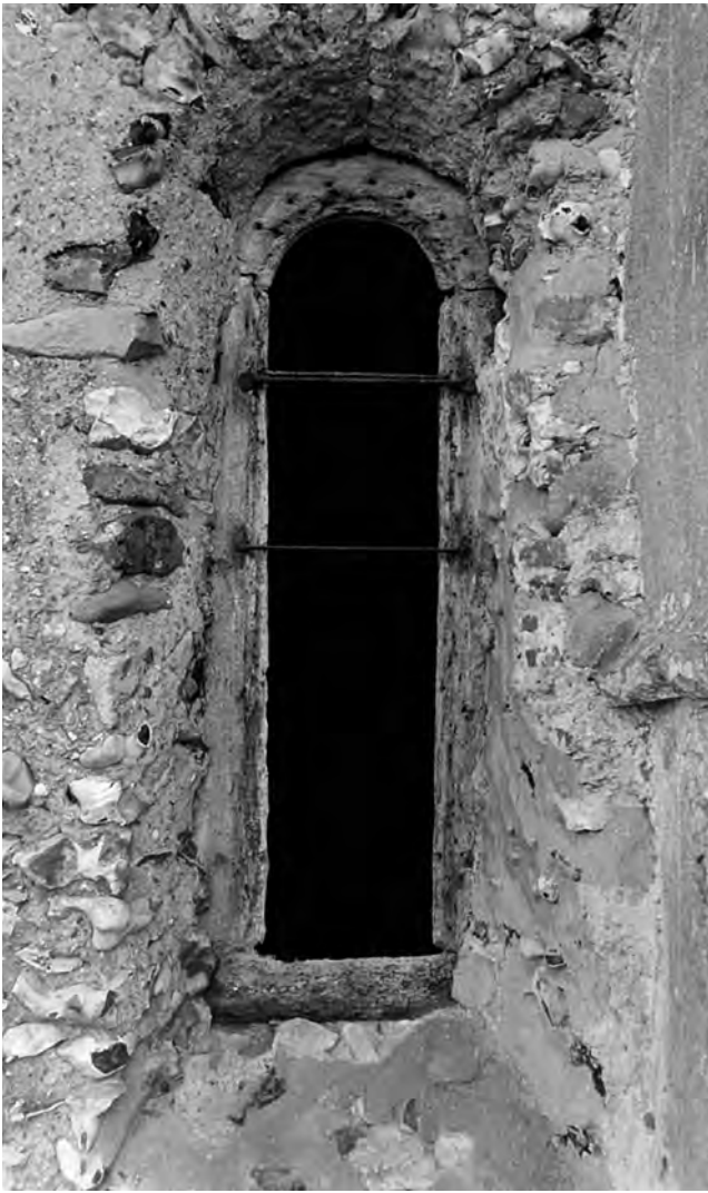
Fig. 331: St Botolph, Hadstock (Essex). Jointed oak frame of a double-splayed window in the north wall of the nave, integrally built with the flint-rubble masonry. Note also remains of the original lime-render in the reveal and on the external wall face (upper left). Photo: Warwick Rodwell
