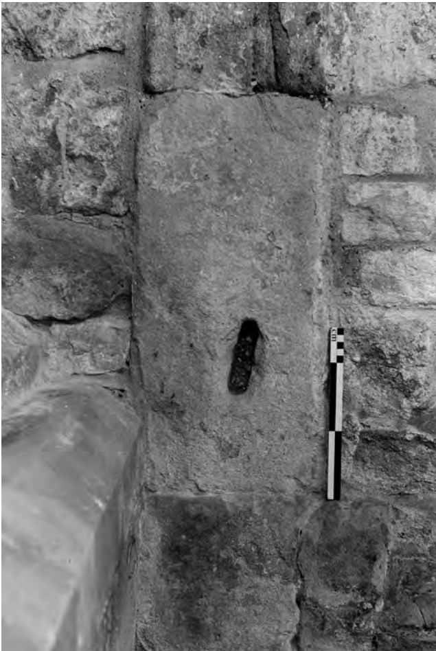
Fig. 362: St Peter, Barton-upon-Humber. Tower: south-east quoin. Lewis hole in the east face of the first upright block of gritstone (now visible inside the nave). Scale of 25 cm. Photo: Warwick Rodwell
