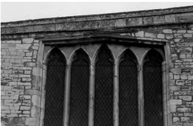
Fig. 56: St Mary's: south chancel aisle. Upper, east end, with its truncated window. Lower, detail of the window tracery and substitute cambered head. Photos: Warwick Rodwell
