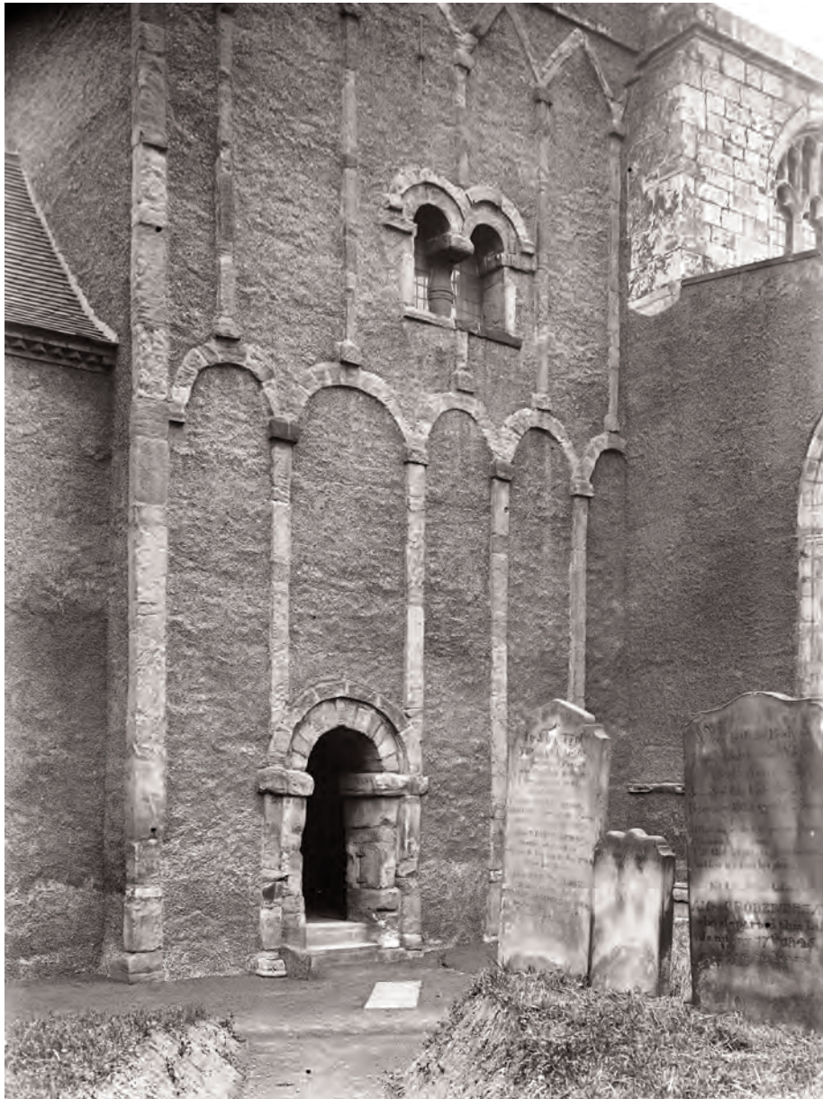
Fig. 610: Roughcast rendering on the tower, western annexe and south aisle, applied in 1868–70. View from the south-west, c. 1900. Photo: English Heritage, NMR
