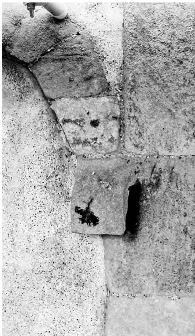
Fig. 263: Tower: Stage 1A, north. Square impost at the west end of the wall arcading. This detail, which is integral with the ashlar of the north-west quoin, projects both laterally and forwards. Note the small, non-radial voussoirs. Photo: Warwick Rodwell
