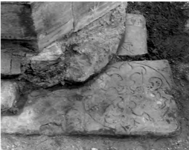
Fig. 484: South arcade. Pier base 2/3, showing the upper end of a grave-cover (F4199) reused in the footing; beyond is glimpsed the lower end of a second grave-cover (F4198). View west. Photo: Warwick Rodwell
