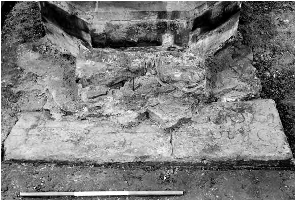
Fig. 485: South arcade, bay 4. Stub of the destroyed arcade bench adjoining pier 4/5. Note the thirteenth-century decorated grave-cover (F4197) reused as a footing for the pier. View west. Scale of 75 cm. Photo: Warwick Rodwell
