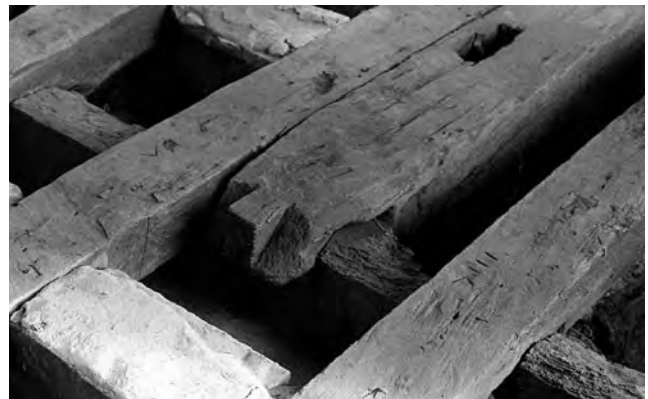
Fig. 547: South porch roof. Detail of reused timber (with mortice on the upper side) at the south-west corner of the roof; view looking north-east. Photo: Warwick Rodwell
