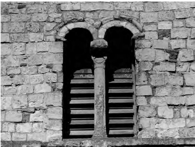
Fig. 405: Tower: Stage 3, south face of belfry. Upper, before restoration in 1965 (note the raised sill and decayed rendering of c. 1870). Lower, in 2000. Photos: David Lee Photography; Warwick Rodwell
