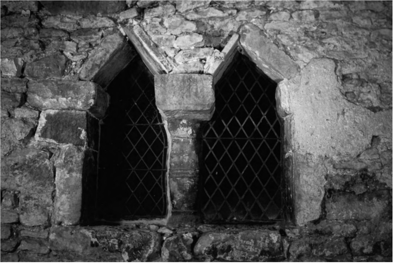
Fig. 297: Tower: Stage 2. South belfry opening with original wallplaster overlapping the right-hand reveal, 1983. Note the nineteenth-century slabs of Yorkstone, replacing original timbers on the two inner slopes of the gabled heads. Photo: Warwick Rodwell
