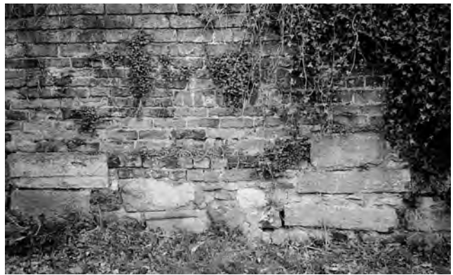
Fig. 42: St Mary's: eastern churchyard wall (c), adjoining the Beck, showing reused moulded stones and flat limestone slabs. Photo: Warwick Rodwell
