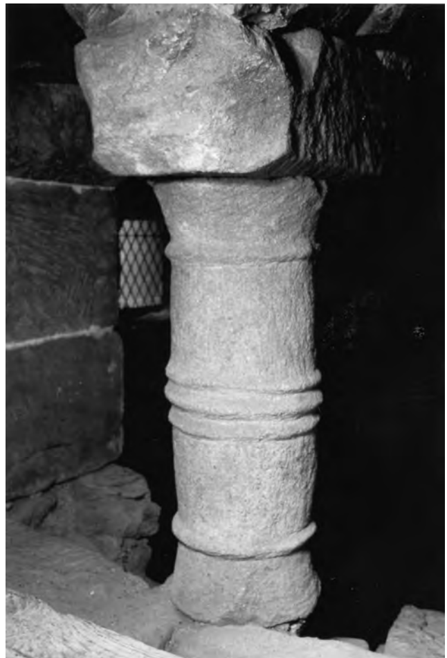
Fig. 314: Tower: Stage 2, exterior. Baluster and through-stone in the eastern belfry opening. View south-west. Photos Figs 313 and 314: Warwick Rodwell
