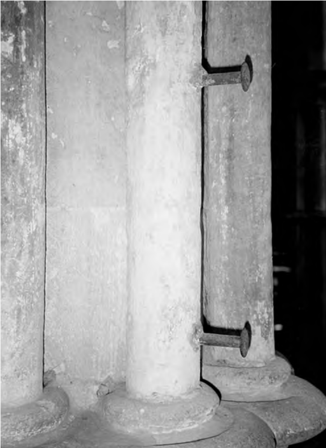
Fig. 72: St Mary's: south nave arcade. Two iron pins set in lead in one of the shafts of the pier between bays 1 and 2. The pins were probably for securing the rope that operated the medieval rood veil. Photo: Warwick Rodwell
