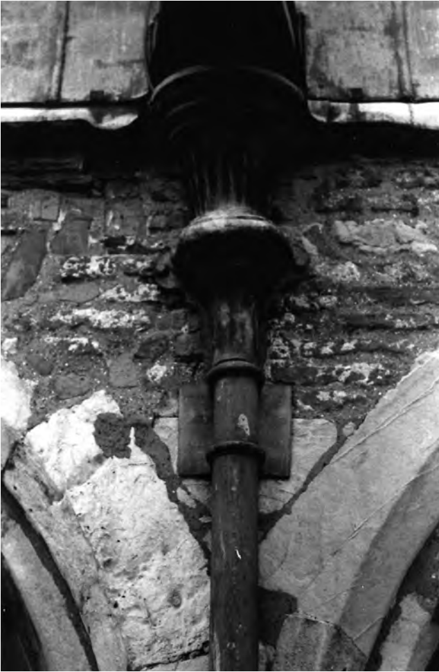
Fig. 585: South clerestory, western rainwater pipe. Fluted lead hopper-head and plain modern downpipe between window bays 8 and 9. Photo: Warwick Rodwell
