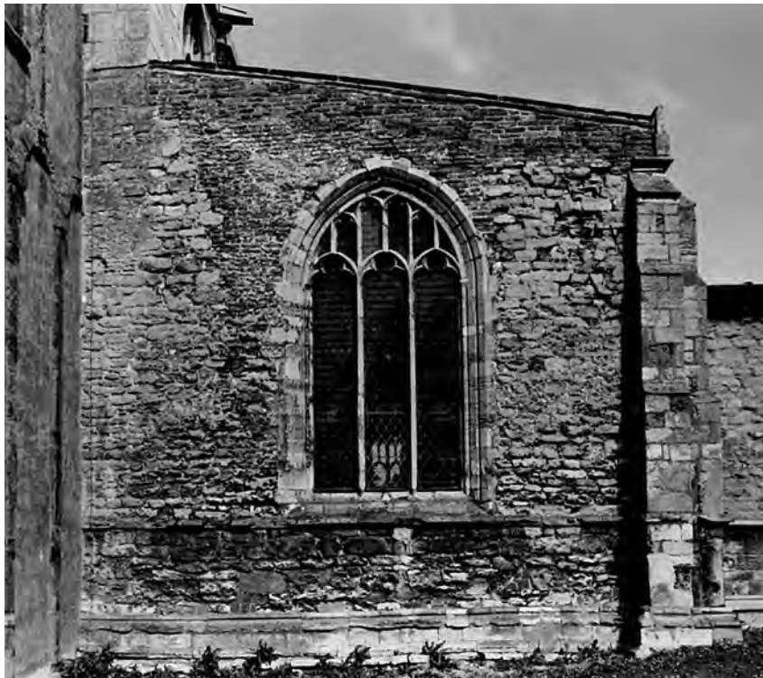
Fig. 545: South aisle. Modified west window, with partial rebuilding of the wall above in brick; unrestored, 1999. Photo: Warwick Rodwell
