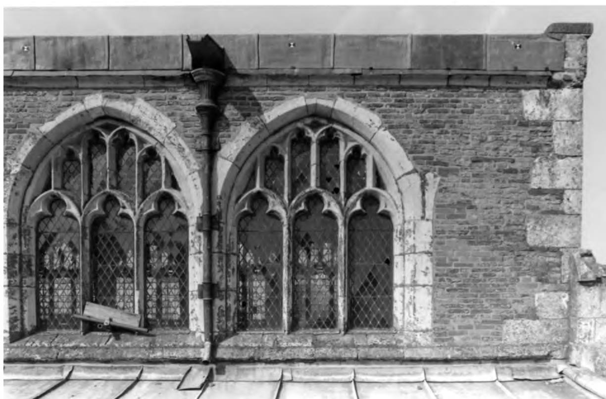
Fig. 543: South clerestory. A, Bay 9 (west); B, Bay 1 (east); showing windows and adjoining nibs of brickwork and ashlar masonry, 1980. Note also the springing for an unbuilt tenth bay to the east. Photos: Warwick Rodwell
