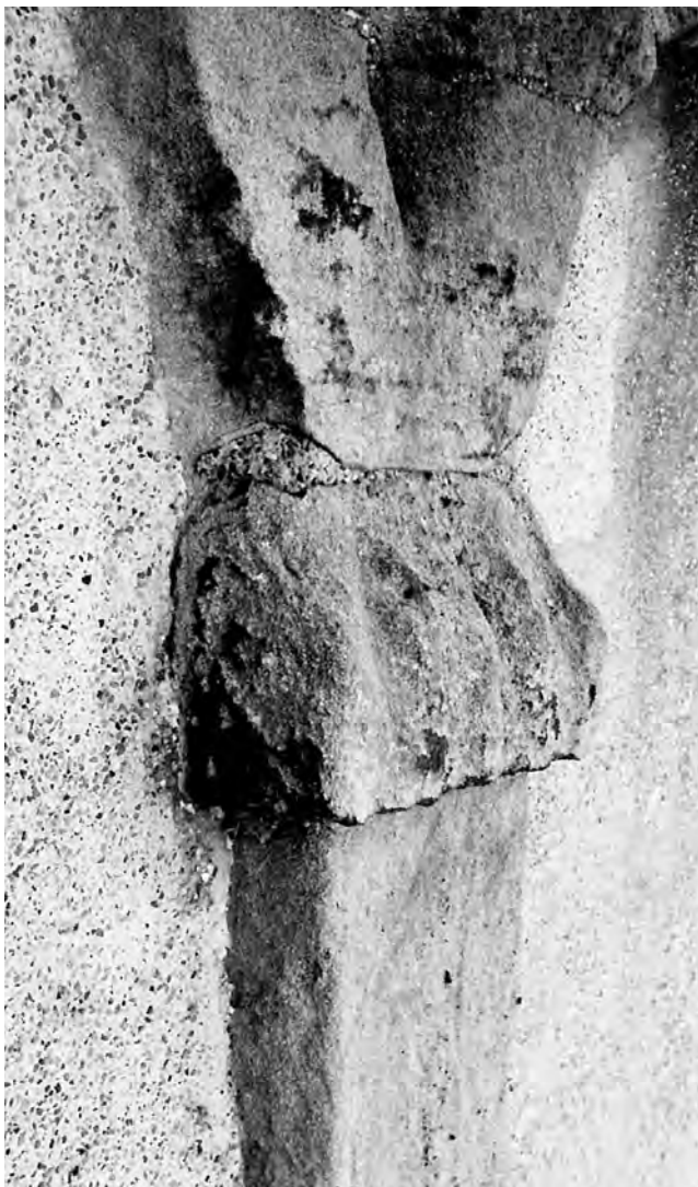
Fig. 262: Tower: Stage 1A, south. Plain rectangular capital, now heavily eroded and giving a false impression of being decoratively fluted. This capital supports the only example of a double-springer at this level which was specially shaped to seat the lowest voussoirs of the adjoining arches. Photo: Warwick Rodwell
