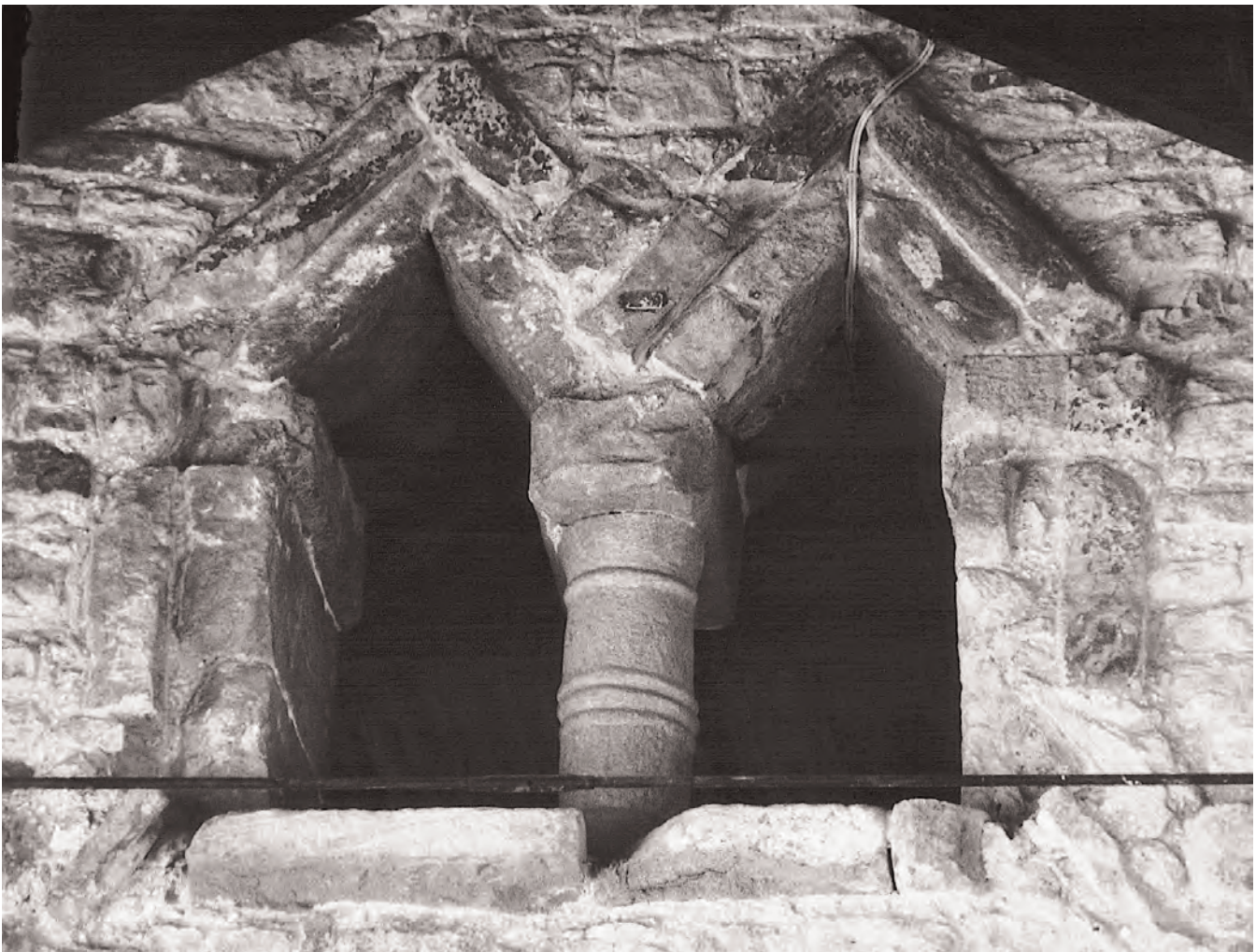
Fig. 276: Tower: Stage 2. East double belfry-opening, seen from within the medieval nave. Note the remains of the head-stops, particularly on the left. See also Fig. 377. Photo: Derek Craig. © Corpus of Anglo-Saxon Stone Sculpture
