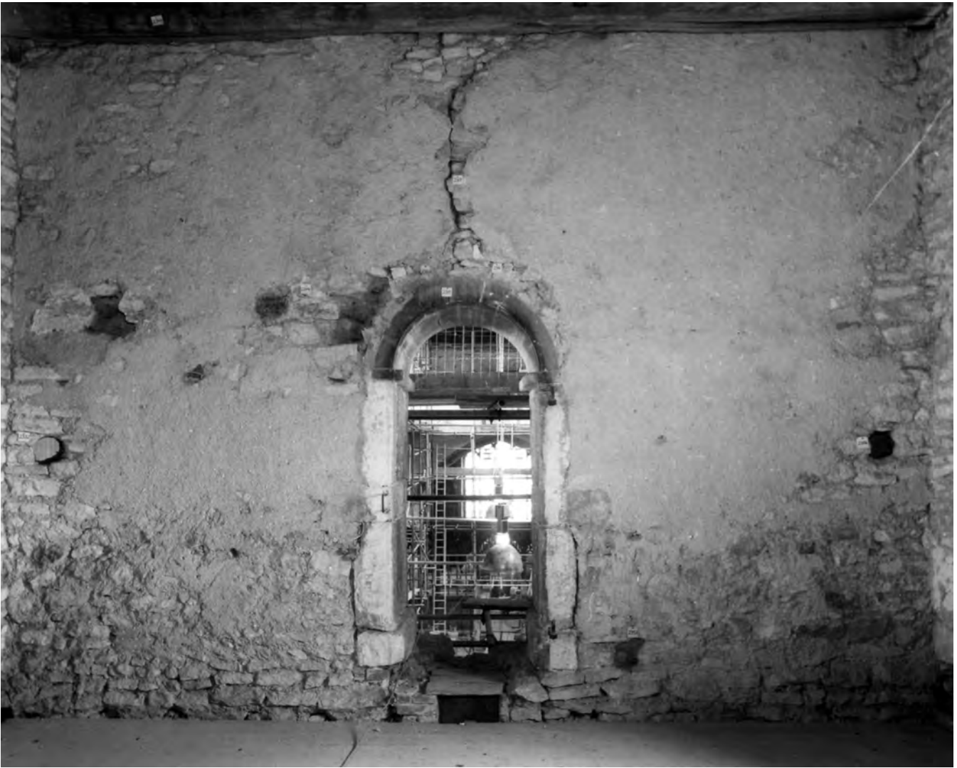
Fig. 290: Tower: Stage 1B, interior. High-level doorway in the east wall (west face), and surviving Anglo-Saxon wall-plaster, 1983. The darker stones comprising the arch date from 1858. Photo: English Heritage Photo Library
