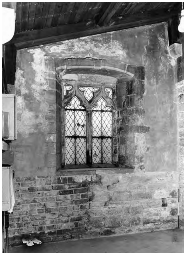
Fig. 537: Vestry. Interior showing the east wall which was partly rebuilt in brick in 1897. Photo: Warwick Rodwell
