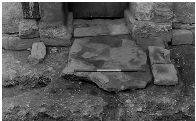
Fig. 419: Tower: south doorway. Step (F3282) and threshold slab (F3035) lying on the Period 2 churchyard surface. Scale of 75 cm. Photo: Warwick Rodwell
