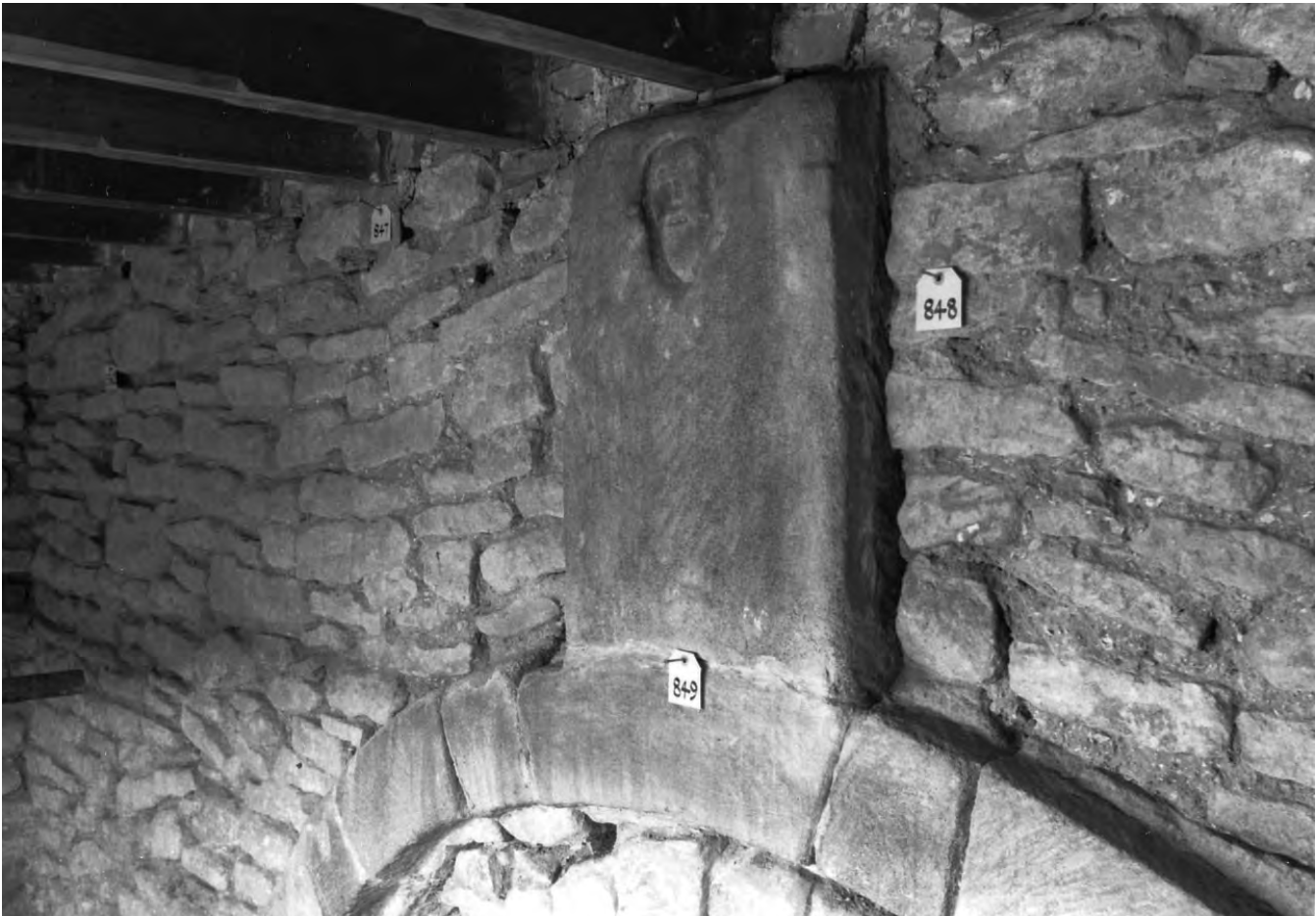
Fig. 309: Tower. 'Humping' of the masonry courses over the eastern arch. View north-east. Photo: Warwick Rodwell
