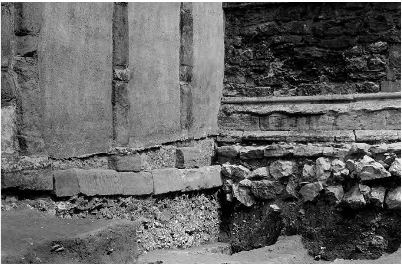
Fig. 264: Tower: plinth and base-blocks of the pilasters, exposed by excavation. These had been buried by the rising churchyard level by the late thirteenth century, when the south aisle (right) was built. Photo: Warwick Rodwell
