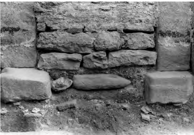
Fig. 421: Tower: north doorway. Period 3 soil and pebble infill, raising the threshold to the level of the respond bases. Photo: Warwick Rodwell
