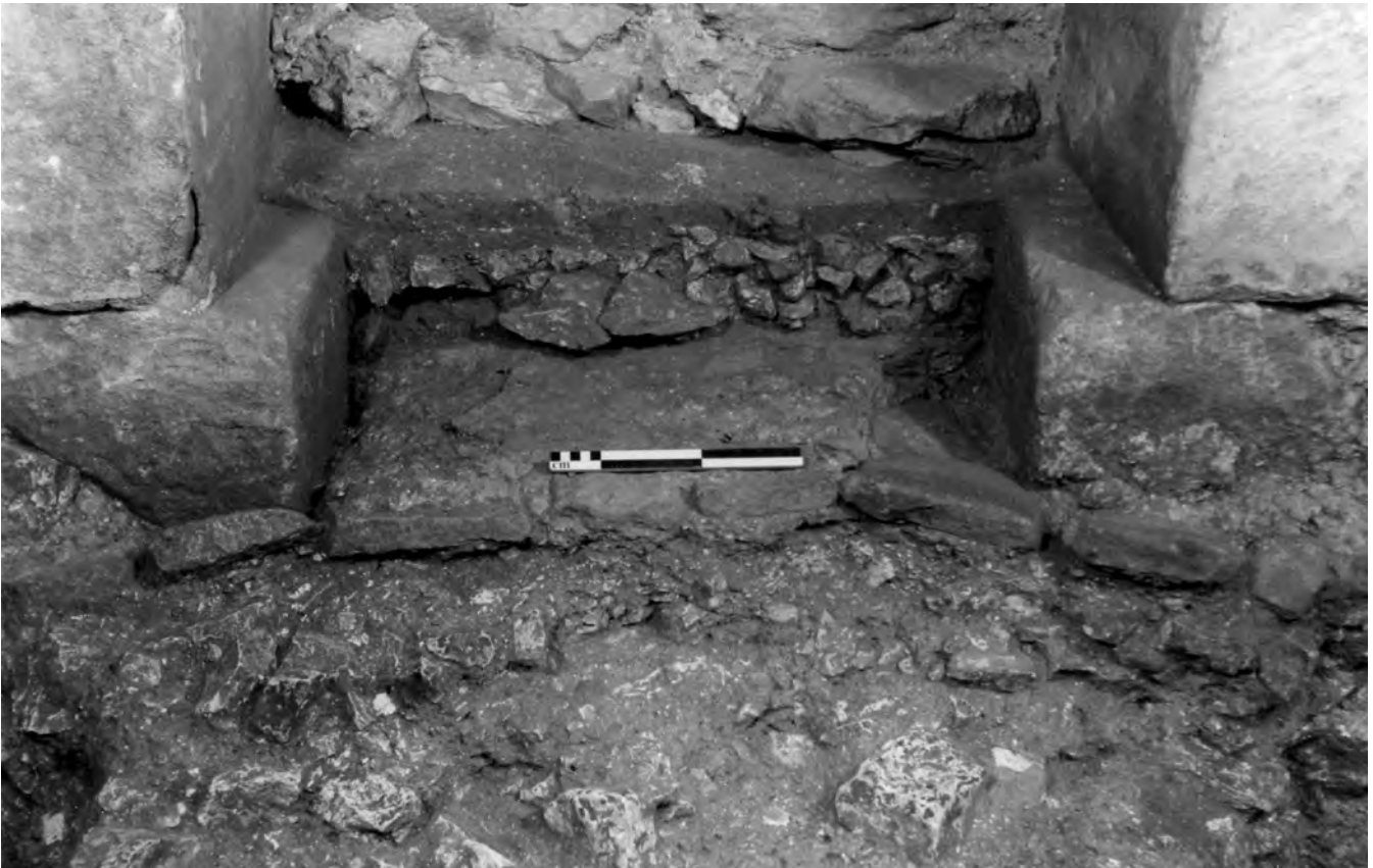
Fig. 316: Tower: threshold of the north doorway. The opening was originally edged with flat pieces of stone and finished with lime concrete; small rubble and a layer of grey loam were deposited over the threshold in Period 5, before the doorway was completely infilled with rubble. View north. Scale of 25 cm. Photo: Warwick Rodwell
