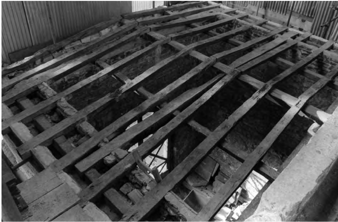
Fig. 546: South porch. View of the roof, from the north-east, after stripping the lead and boarding, 1983. Photo: Warwick Rodwell
