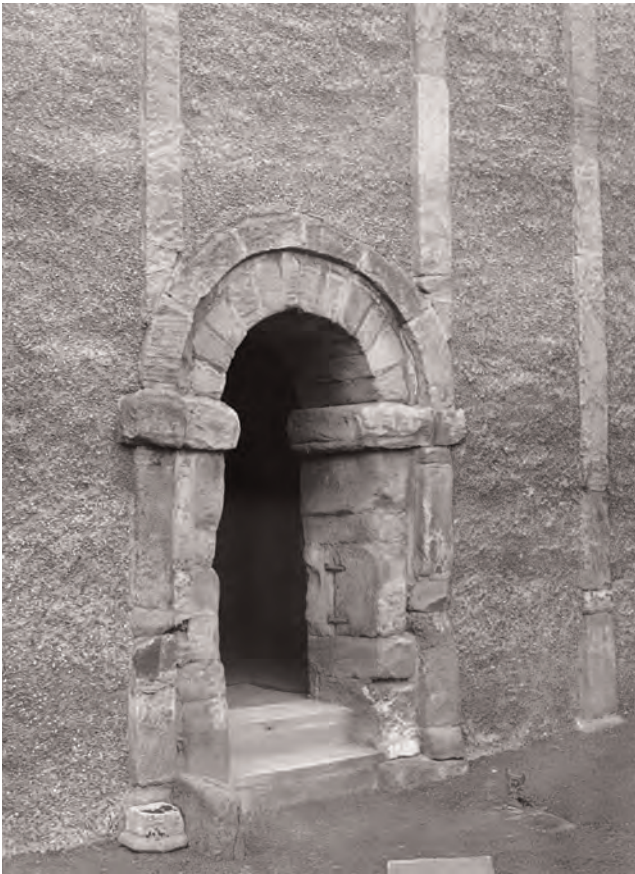
Fig. 266: Tower: south doorway, c. 1900. Taken before internal floor level was lowered and the steps removed. This also shows the pebbledash rendering that was applied c. 1870. Photo: English Heritage, NMR
