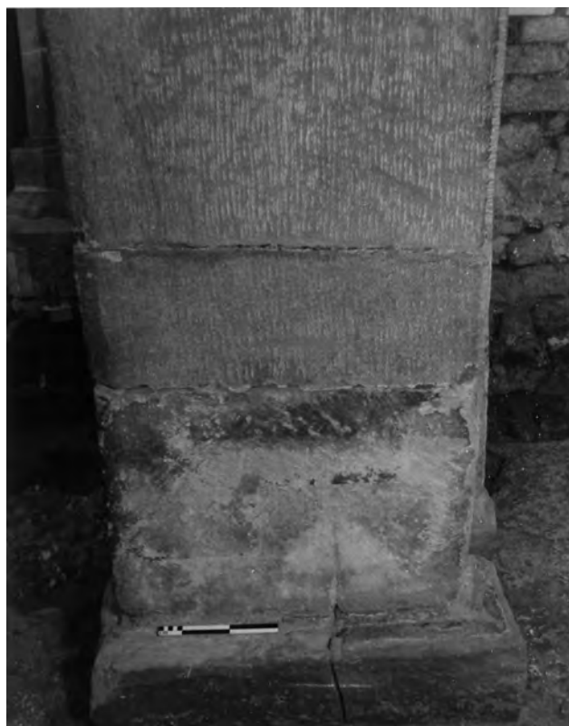
Fig. 281: Tower: Stage 1A, eastern arch. A, north, and B, south responds and bases, showing settlement fractures and Victorian redressing of the masonry (vertical clawing). Scale of 25 cm. Photos: Warwick Rodwell
