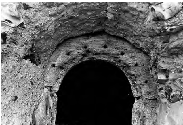
Fig. 332: St Botolph, Hadstock (Essex). Semicircular head of a jointed window frame in the nave, showing the arc of small holes used to anchor the basketwork hood which served as a former for the arch of flint rubble. Note the preserved wattle impressions in the soffit. Photo: Warwick Rodwell
