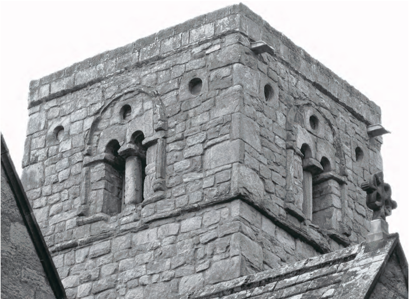
Fig. 293: St Andrew, Bywell (Northumb.). Semicircular heads of the double belfry openings formed from rectangular blocks of Roman masonry, possibly reused window heads. Photo: Warwick Rodwell
