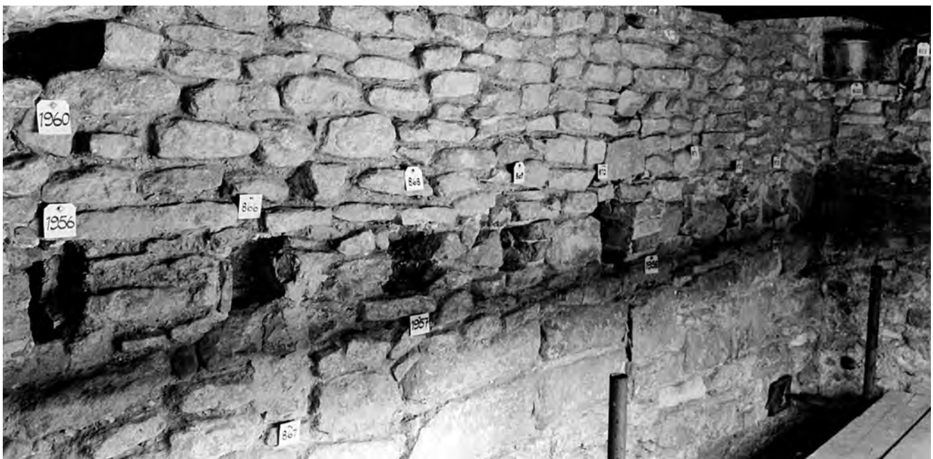
Fig. 579: Tower, south wall. A series of pockets cut to receive the joists for a post-medieval ringing-chamber floor which was removed again in 1858. Note the stone corner-bowl at top right (see Fig. 580). View south-west, 1980. Photo: Warwick Rodwell
