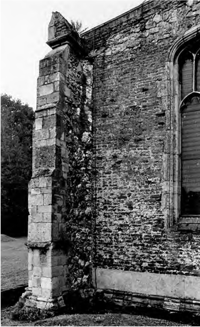
Fig. 562: South aisle. Detail of the south-east clasping buttress, showing how the Tudor east wall was set further west than its predecessor, leaving a rubble scar on the side of the buttress. Photo: Warwick Rodwell
