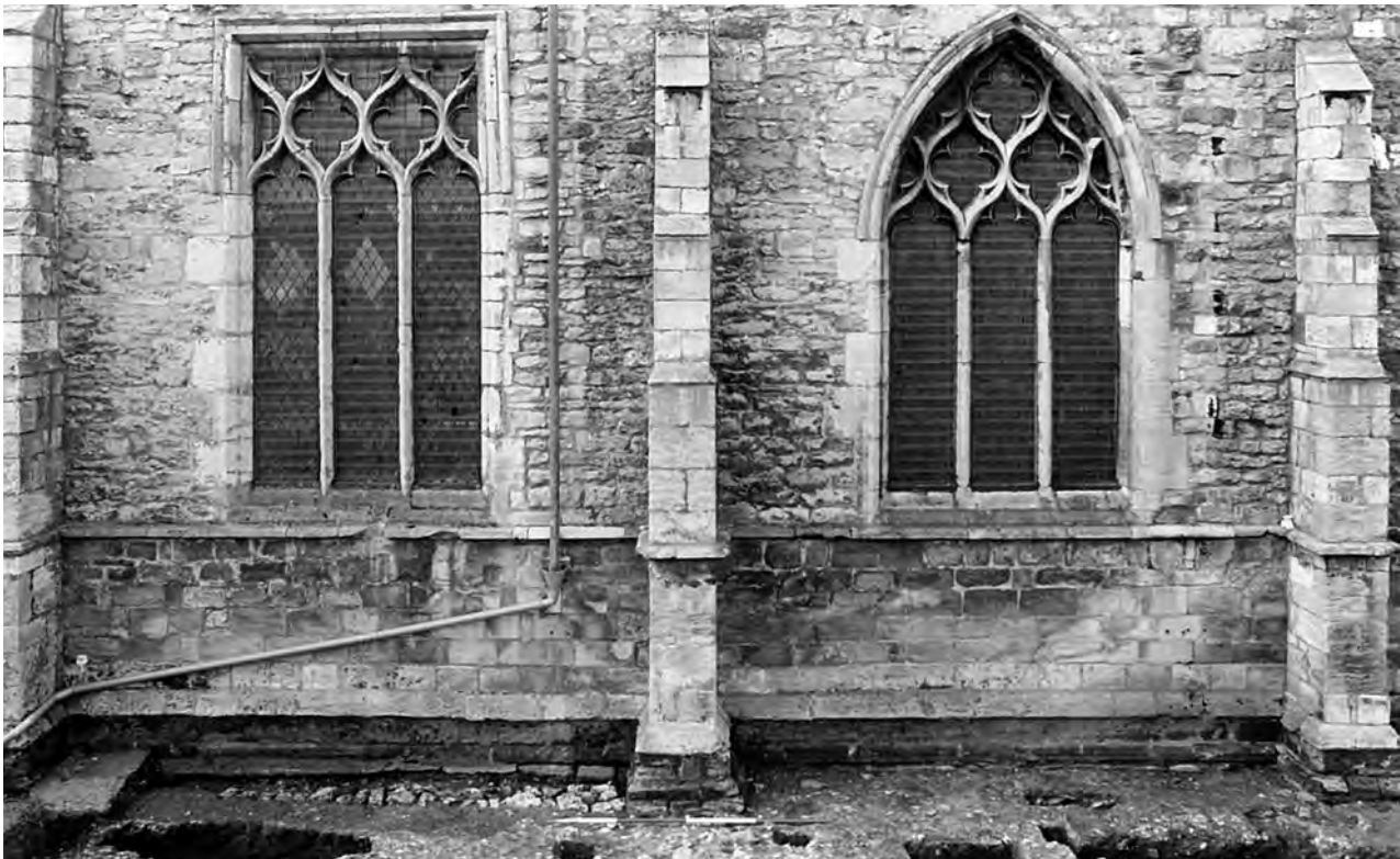
Fig. 468: North aisle windows, bays 1 and 2. The windows have reticulated tracery, and are alternately square-headed and pointed. Contemporary construction level for the aisle has been exposed by excavation externally, 1982. Scale of 2 m. Photo: Warwick Rodwell
