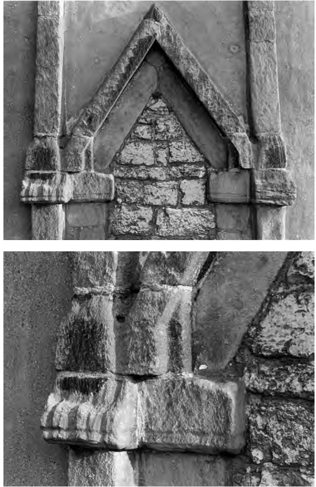
Fig. 271: Tower: north doorway. A (upper), the triangular head. B (lower), construction detail of the eastern impost. Photos: Warwick Rodwell
