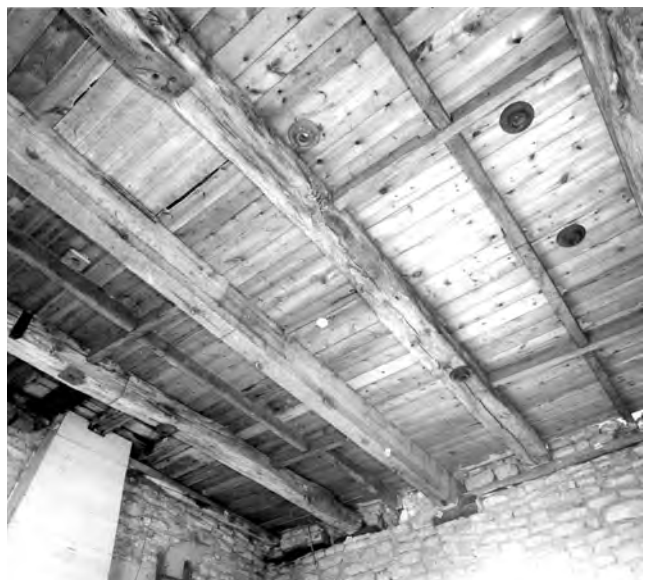
Fig. 295: Tower: floor between Stages 1B and 2. The joists are medieval and later, but the thin spreader-plate in the north wall (right), upon which their ends rest, is primary Anglo-Saxon. Also partly visible on the west side is the casing of the clock pendulum (1852). View north-west, 1983. Photo: English Heritage
